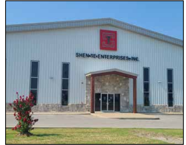
POLSON INDUSTRIAL PARK DEVELOPMENT 49TH W. AVENUE
